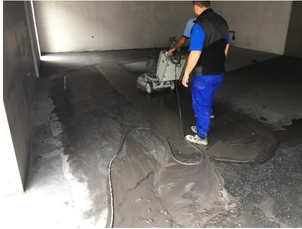
Figure 6 Wet Diamond Grinding & Resin Pad Application
