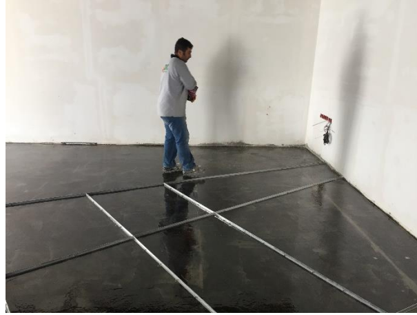
Figure 3 Sanding after Epoxy Primer Application
