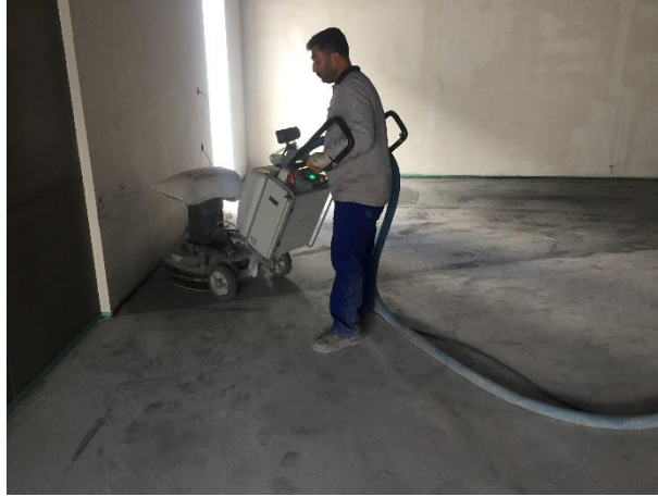
Figure 5 Dry Diamond Grinding Application
