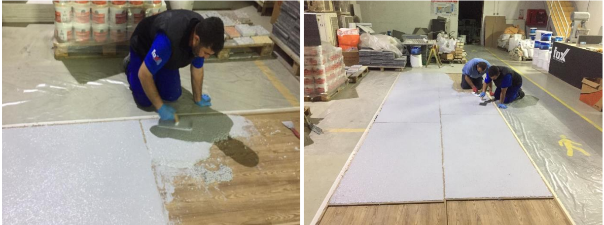
Figure 4 Fox Epothane Basecoat Terrazzo Application
