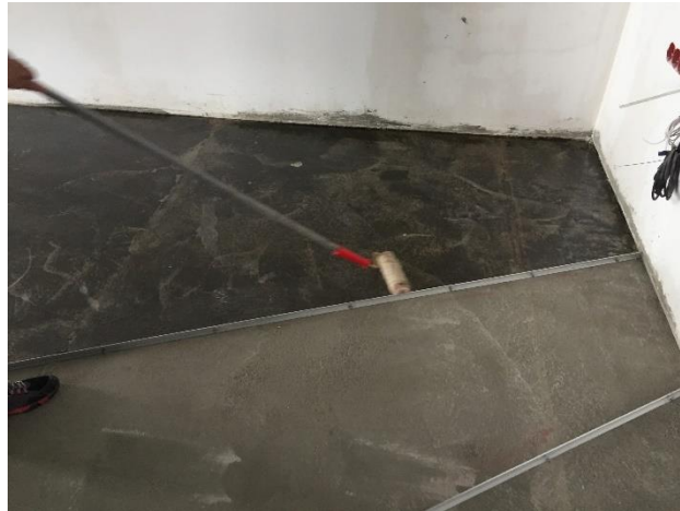
Figure 2 Epoxy Primer Application
